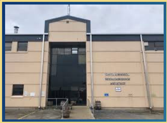
Mendenhall Treatment Plant (MTP)
