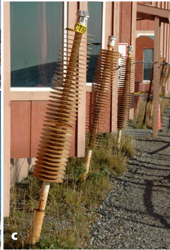
(a) Geodesic dome at Thule Air Base, Greenland. (b) Red Dog Mine port facility, Alaska. (c) Thermosiphons, Kotzebue, Alaska.
