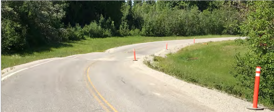
(U) Figure 9. Undulations in the Road Near the Entrance to the Eielson AFB Ammunition Supply Point (U) Source: The DoD OIG.
